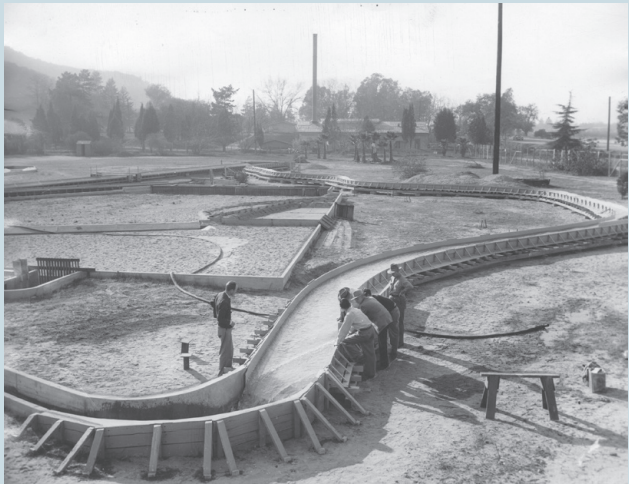
Miniature physical models of the Los Angeles River and other flood control and channel improvement projects in the area, 1948 Photo: Herald-Examiner Collection, Los Angeles Public Library
