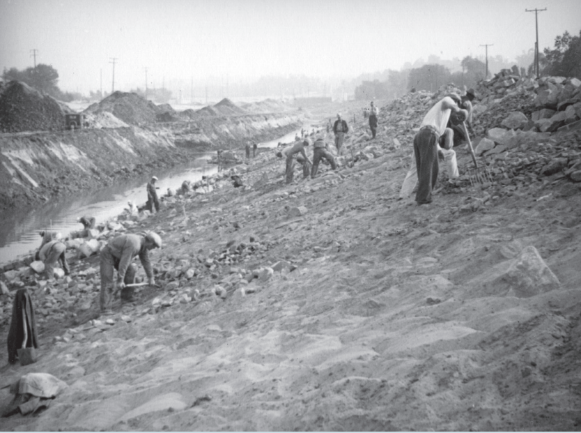
Men remove rocks and boulders from one bank of the Los Angeles River using their hands and rakes during construction, 1938 Photo: Herman J. Schultheis Collection, Los Angeles Public Library
